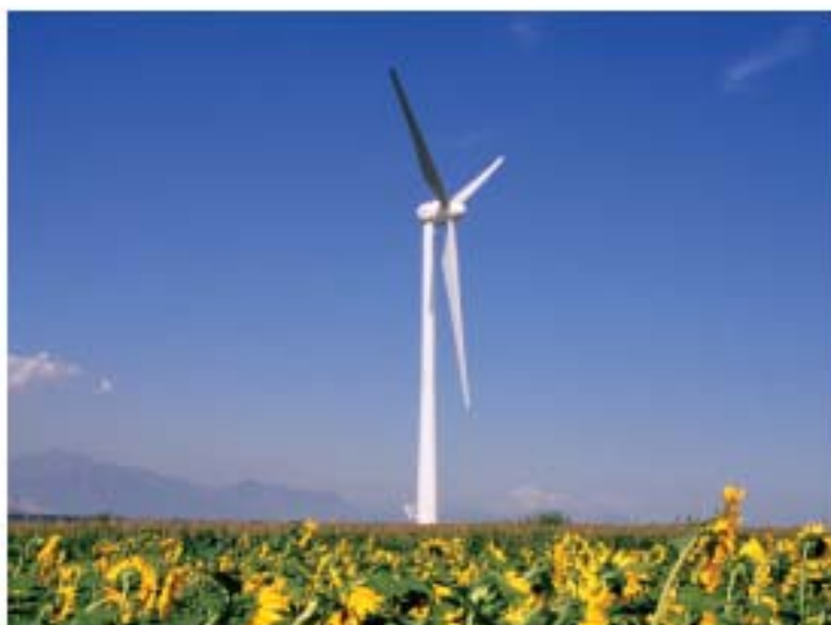
Photo: Goldwind 1.5 MW DD Turbines in Guanting Wind Power Project near to Beijing. James Gavin J.
